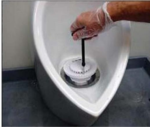
PULL UPWARD ON INSERT TO REMOVE.
