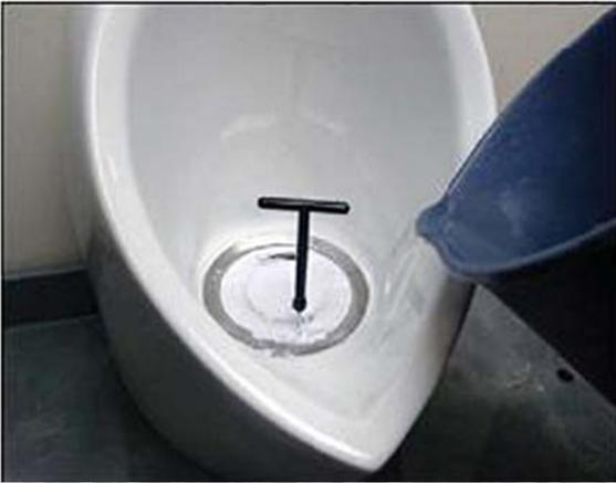
USING THE KEY PROVIDED, SCREW THE KEY INTO THE KEY HOLE OF THE DRAIN INSERT AND FILL WITH WATER
